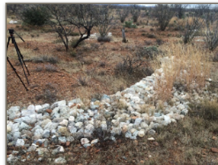
From left to right: Gabion, wire enclosure rock structure in channel; Check dam, loose rock structure in channel; Media luna, loose rock structure on floodplain. Photos credit: Natalie Wilson
