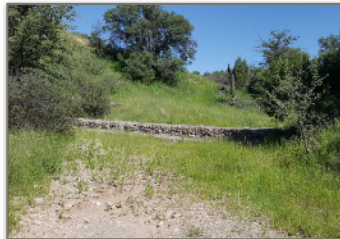
From left to right: Gabion, wire enclosure rock structure in channel; Check dam, loose rock structure in channel; Media luna, loose rock structure on floodplain. Photos credit: Natalie Wilson
