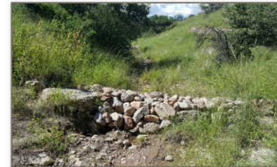
From left to right: Gabion, wire enclosure rock structure in channel; Check dam, loose rock structure in channel; Media luna, loose rock structure on floodplain. Photos credit: Natalie Wilson
